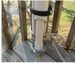
(Pic right) View of the TN three inch 'Lazy Susan' awaiting the attachment of a compass rose. The 'Lazy Susan', being of metal construction with steel ball bearings, when exposed to the elements for extended periods is prone to rust. However for both of the units in NJ and TN after almost a year in use and through all kinds of weather, it has been found that the corrosion can be controlled by liberal periodic application of WD40 or light machine oil.
