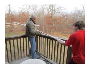
(Pic left) Hinged base of tower permits it to be tilted over to load or remove an antenna by withdrawing or inserting the antenna pipe into the 2 inch diameter outer pipe.
